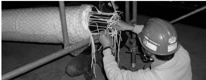
Figure 10. Rigger attaching tie cords to tube end on elevated screen
